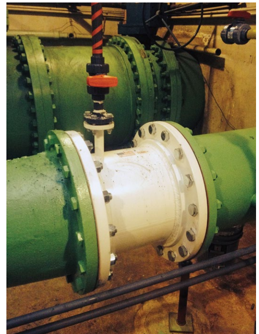
The versatility of Kenics static mixers allows customers to design around existing pipe layout
