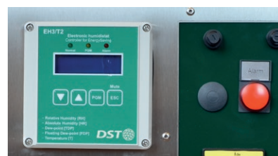
EH3 T2 mounted in a R-61R dehumidifier
