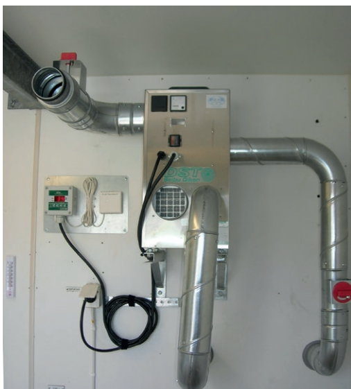
A DR-010B with DST humidistat EH4 controls moisture at a water booster station
